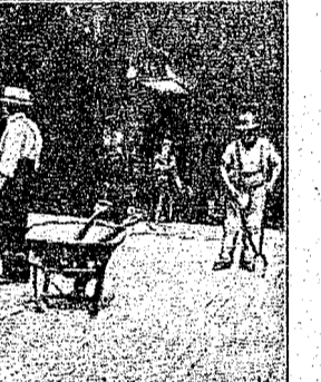
Granite Blocks Laid and Rammed—Maintenance Cost of This Kind of Pavement Is Less Than That of Any Other Kind.
